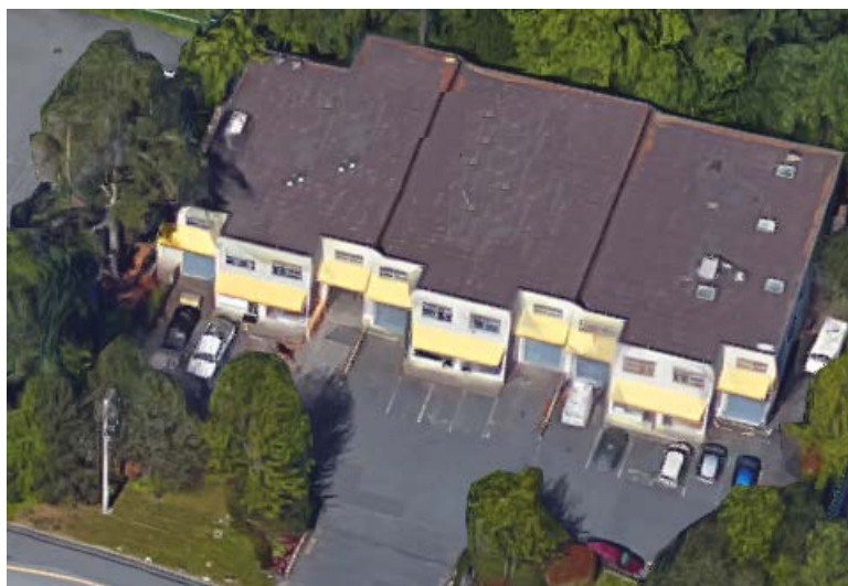
Figure 5 - EMH Facility Overhead View
